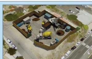
Shaft Site and Staging Area
